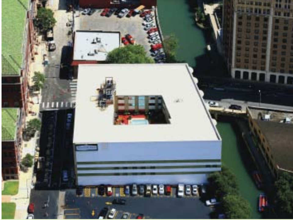
Riverwalk Plaza Hotel San Antonio, TX
